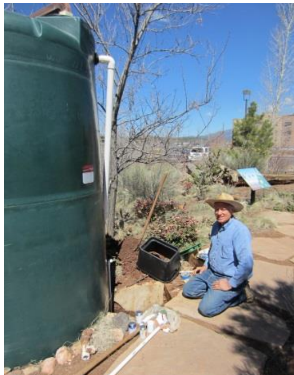
CNRCD Supervisor Norm Lowe installs freeze protection valve boxes for our large rainwater tanks. The rainwater catchment system is used to irrigate our crop garden (see page 7).
