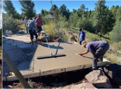
Finishing the Concrete
